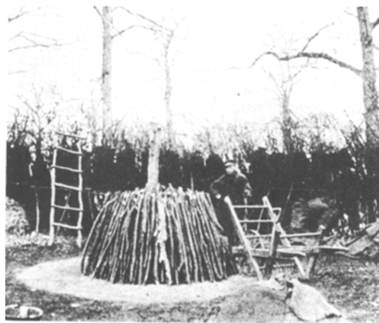
Figure 8 Photograph showing wood stacked around hearth prior to burning [8].
