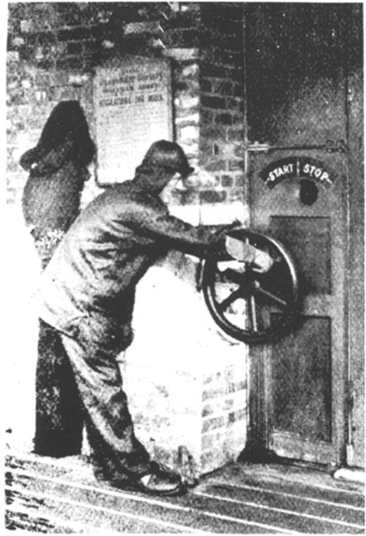
Figure 21 Workers in protective clothing starting incorporating mills [13].
